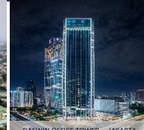
DASWIN OFFICE TOWER - JAKARTA (JO PROJECT)
